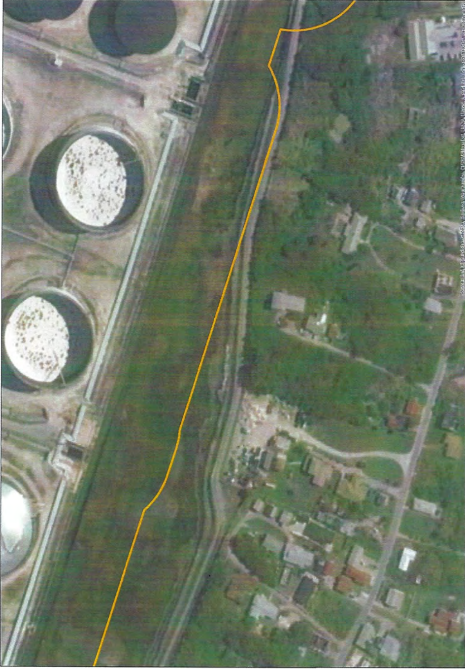
Figure A4.4 The safety buffer zone border at the south-side of Buckeye Bahamas Hub, zoomed in part 3 of 5.
