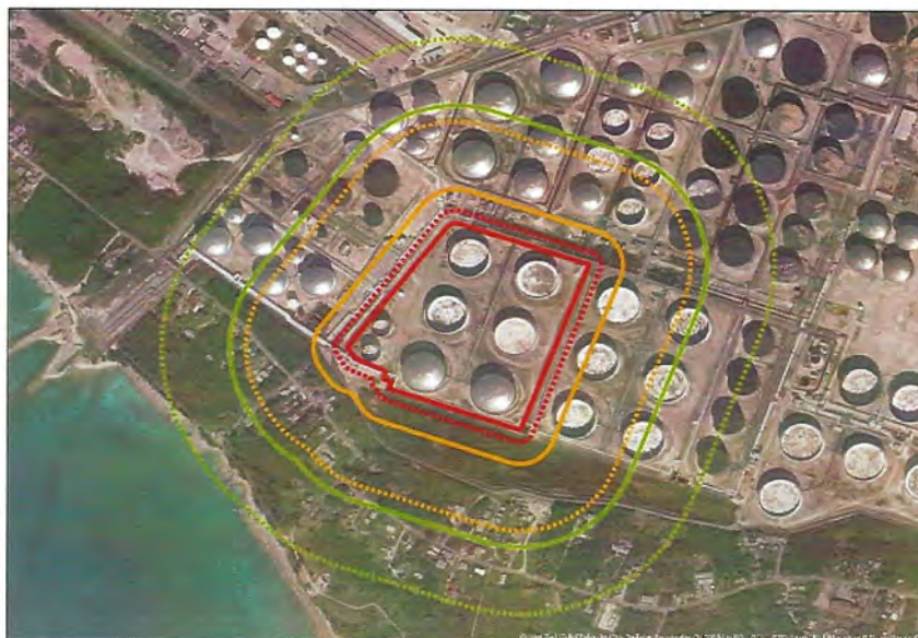
Figure A3.6 Effect distance of scenario 4.6 'Heavy fuel – tank pit (pool size 370 m x 370 m) fire'.
