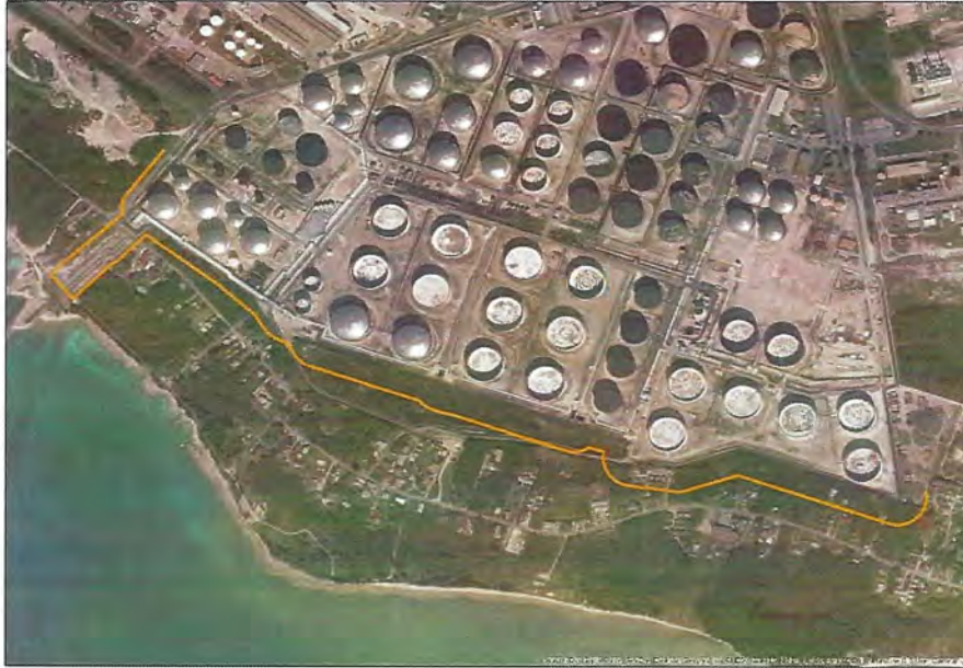
Figure 1.1 The safety buffer zone border at the south-side of the border of Buckeye Bahamas Hub, smoothed out.
