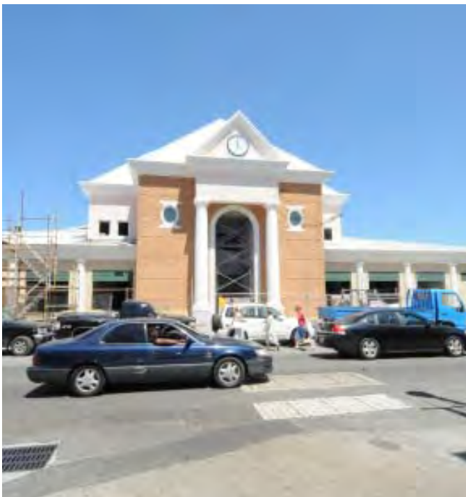
Straw Market, Bay Stret, Nassau. (Under construction)
