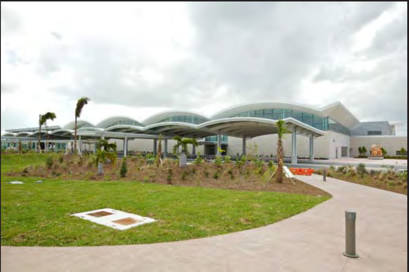
New U.S. Departure Terminal at the Lynden Pindling International Airport (LPIA)
